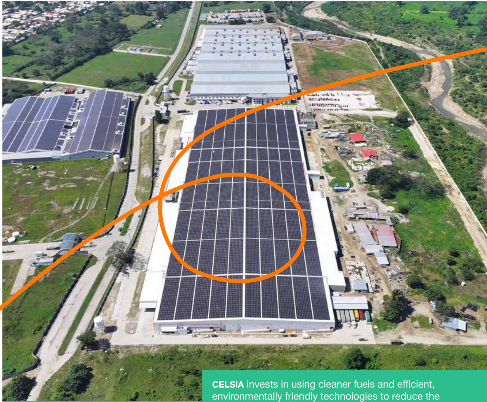
Solar panels in Parkdale Mills Greenfield in Honduras.
