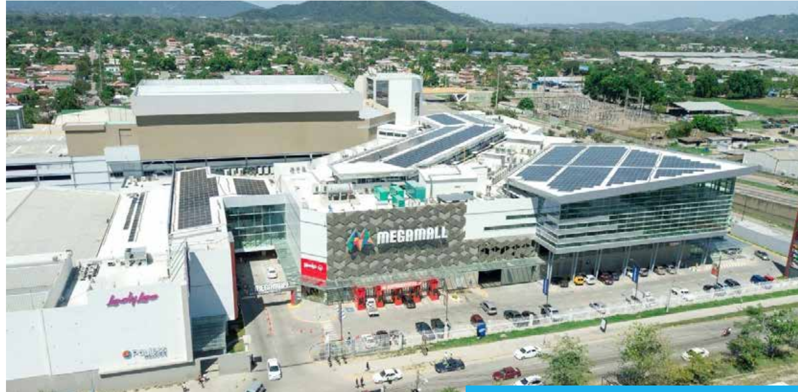
Solar panels in the MegaMall Shopping Center in Honduras.
