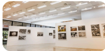
Efficient lighting project - Sura
